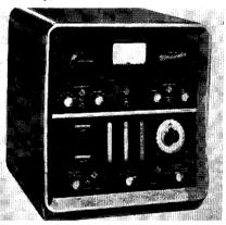
All-purpose scaler for operation with Geiger, scintillation or proportional counters is available from Nuclear Instrument and Chemical Corporation. The instrument, known as the Model 192 "Ultrascaler," permits either manual or automatic counting procedures including either predetermined time or count operation or "time-count" operation where the count will be stopped at a preset time or preset number of counts
